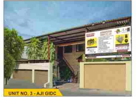
UNIT NO. 3 - AJI GIDC
